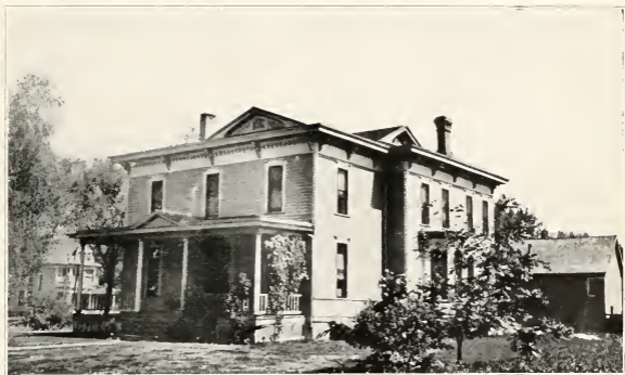
CITY HOSPITAL, GRINNELL
